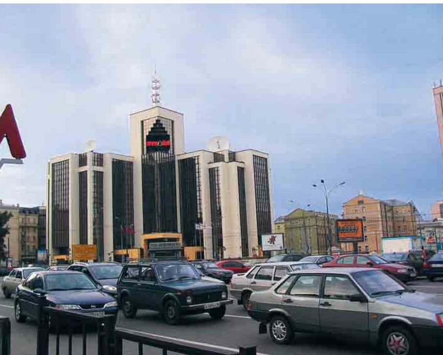
FIGURE 4.28 Moscow, Russia. New office building for LUKOIL, financed by profits generated from high oil prices brought about by recent global demand. Notice expensive cars in foreground parking lot. Photo: © M. Blinnikov.
